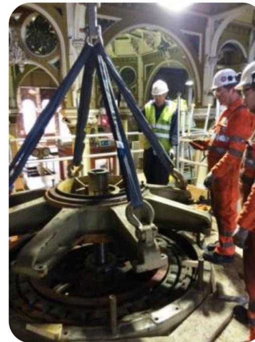
G&G - Removal of a Ø2m Motor Assembly
